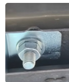
3 Install the metal washer + nut
